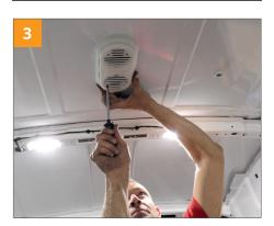
Screw the cover plate onto the inside of the roof using the screws provided. The roof fan is installed: easy!
