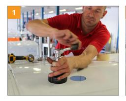
Mark out the holes using the drilling tem-plate provided and create the holes in the roof using a 90 mm punch (available upon request).
