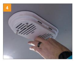
Step 4 is only needed when installing an existing VanFan, as this cover plate is only used for the mechanical version. Detach the screw part (unclick). Unscrew four screws and remove the cover plate.
